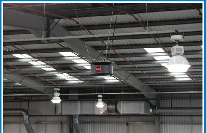
The system uses a high pressure pump to run water through flexible pipework at high level, well out of the way of production, which branches off into sections of the production area and produces a fine mist over target areas.
