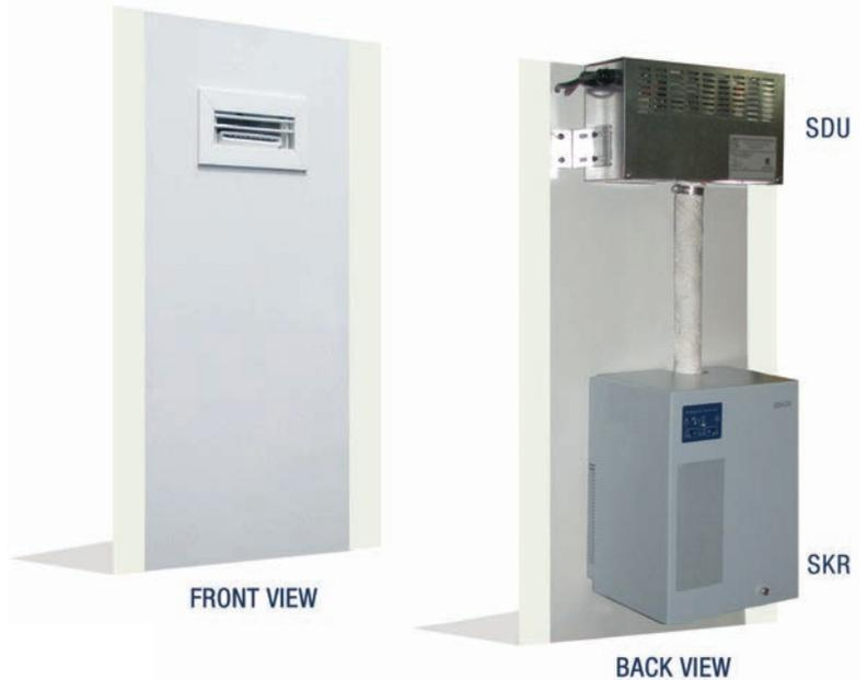
The Neptronic SKR Steam Humidifier with through wall duct.
