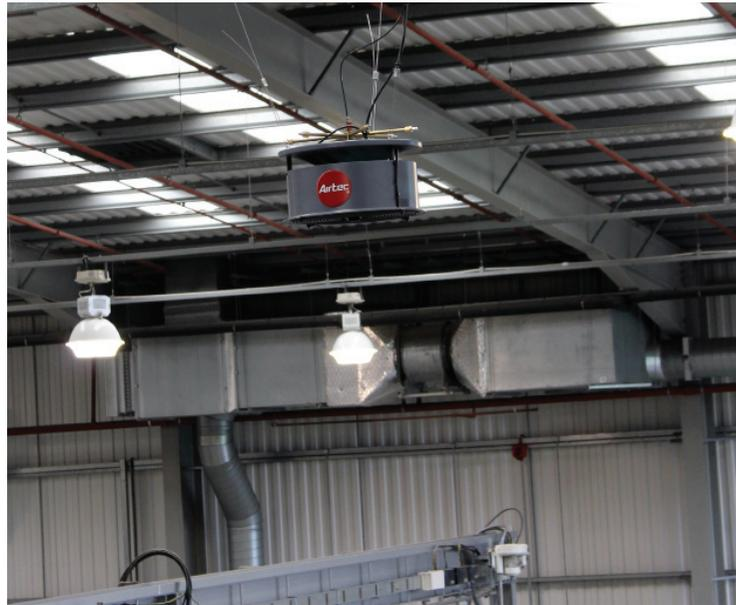
In some situations the most suitable option is to retrofit an evaporative humidifier into an existing air duct system, assuming that the key design criteria can be satisfied. For example, it is important to ensure a very short evaporative distance from the humidifier to avoid condensation or wetting in the air handling unit and the ductwork.
