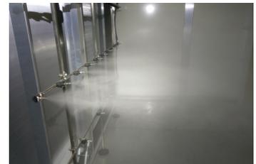
Airtec Hydrosens high pressure water humidifier providing humidity control and adiabatic cooling
