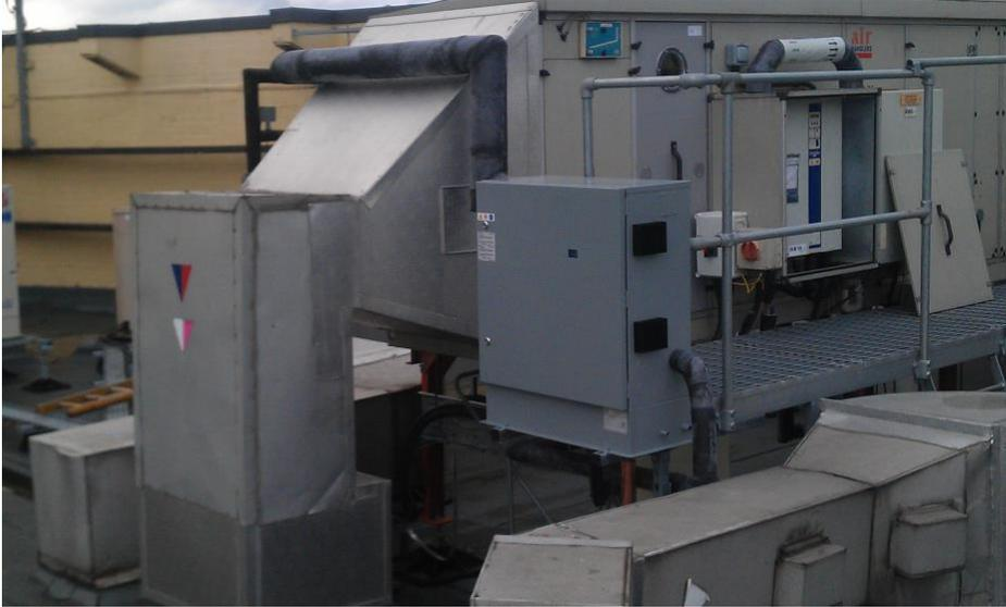
Picture 3 shows the neatness of the weatherproof humidifier (Mounted at the end of the walkway) and the humidifier within a weatherproof housing (with door off to the right of the AHU access panel).
